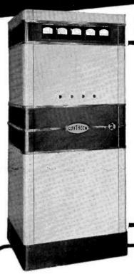
250 Watt FM Transmitter, also standard exciter unit for all higher power.
